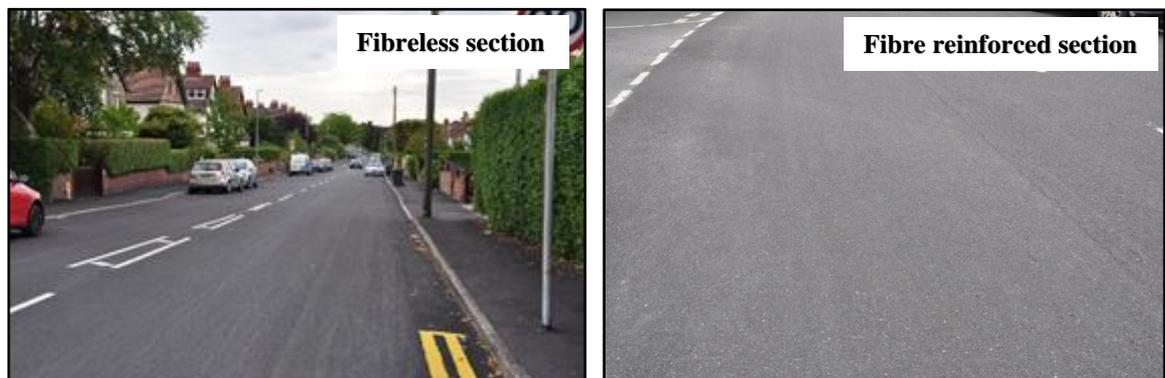
**Figure 7-12: Condition of Talbot Road on inspection at 12 months, fibreless section on left and a closer look at the surface texture of fibre reinforced section on right**
