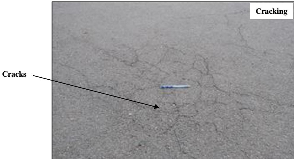
**Figure 7-3: Myriad of extensive cracks**
