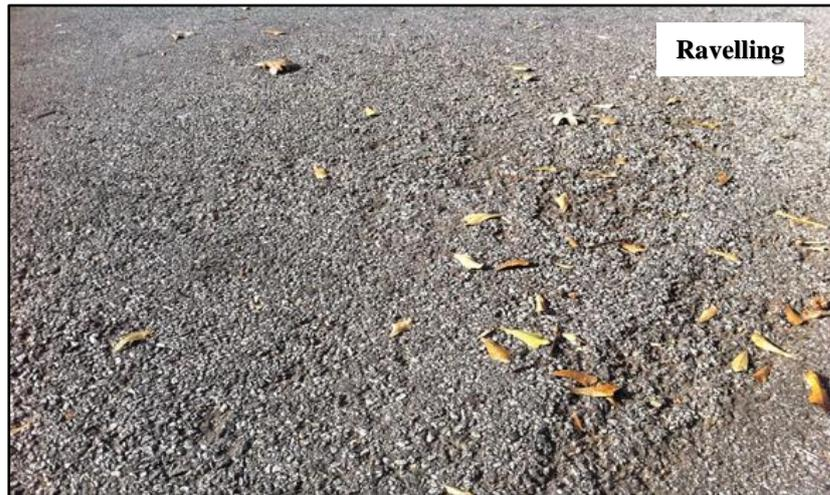
**Figure 5-9: Ravelling in asphalt concrete pavement**
