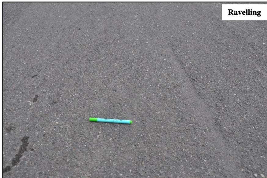
**Figure 7-17: Minor ravelling in fibreless section**
