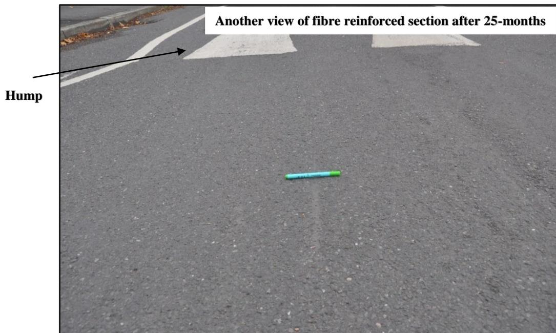
**Figure 7-19: Glass fibre reinforced section near hump**
