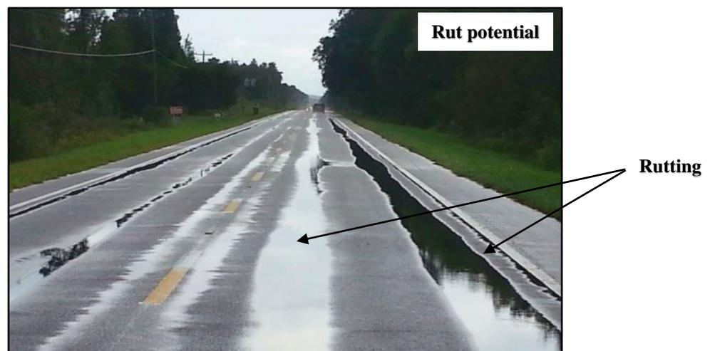
**Figure 5-8: Rutting in asphalt concrete pavement**
