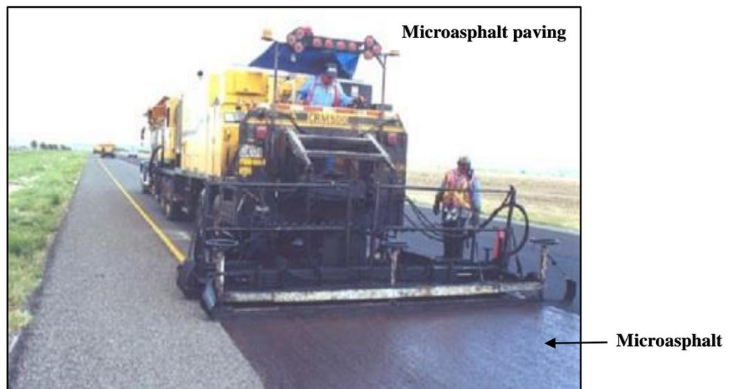
**Figure 4-4: Machine laying microasphalt on site**
