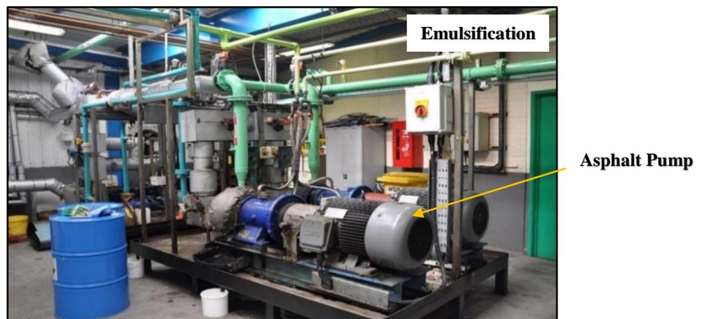
**Figure 5-18: Emulsification of bitumen emulsion in progress**
