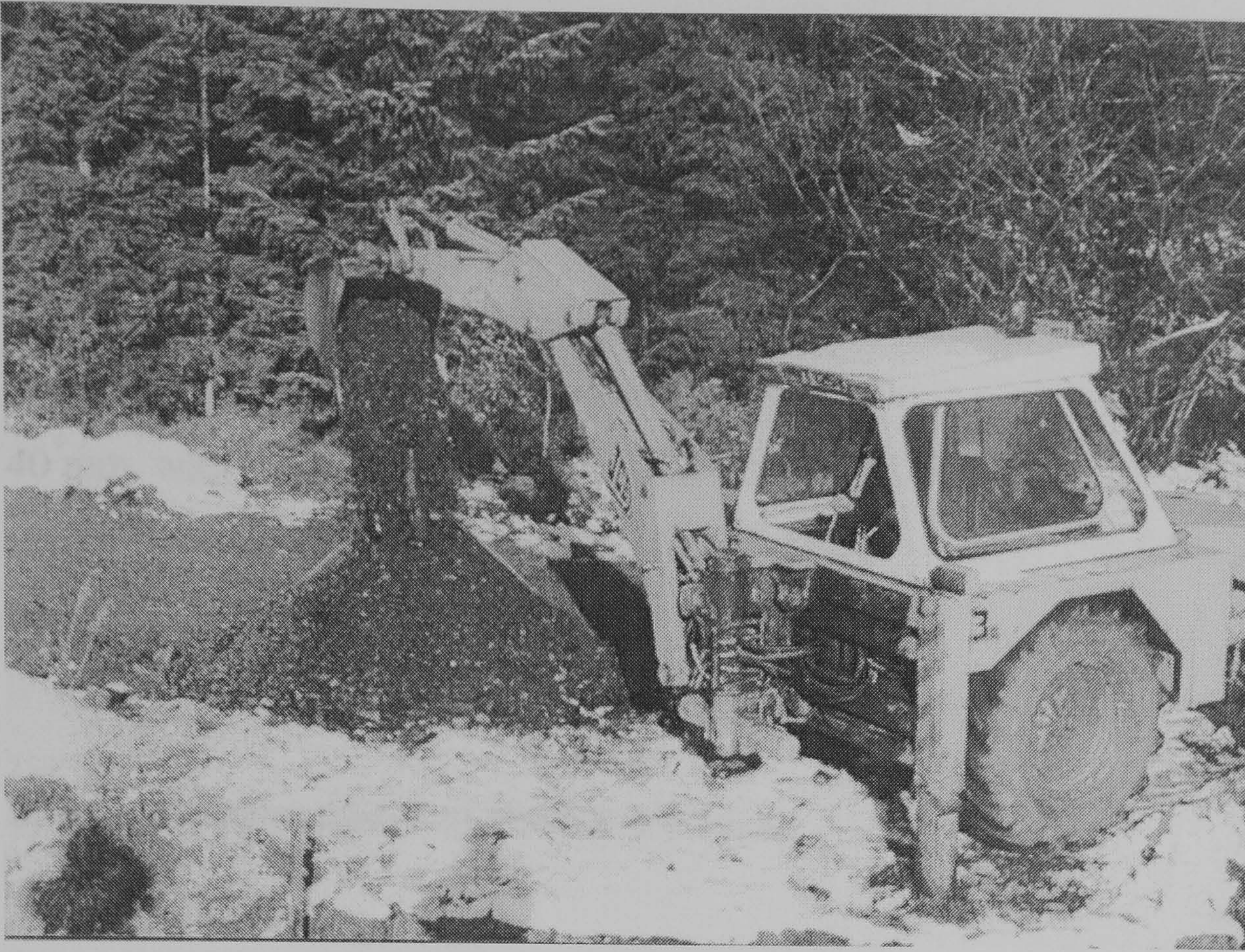
Plate 3.3. Nant Tanllwyth bedload trap: JCB excavation onto measuring spike.
