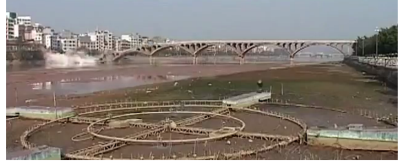
Figure 1: In (a) the demolition of a bridge Guangxi, China. The excavator in this picture was used to initiate some failure at one end of the bridge propagates through the structure. The figure shows the resulting periodic failure process, where the supporting columns fail sequentially causing the collapse of the bridge. An alternative view of this process is presented in (b).
